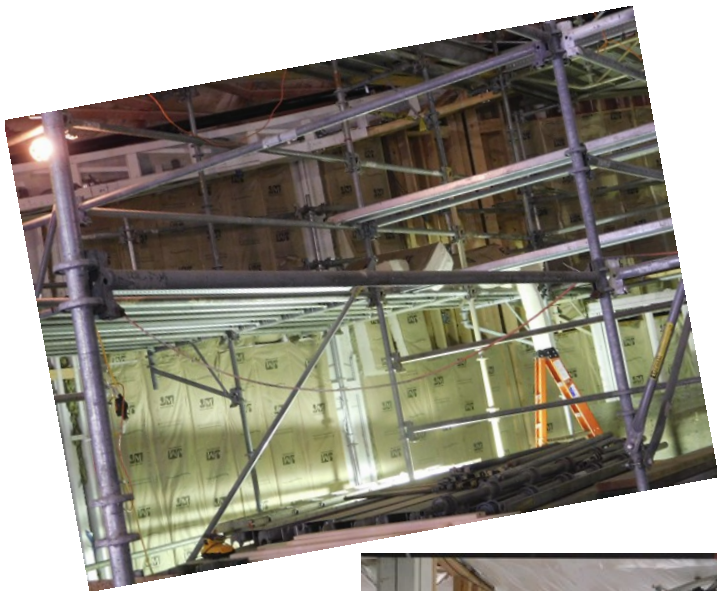
Insulation in the Sanctuary
