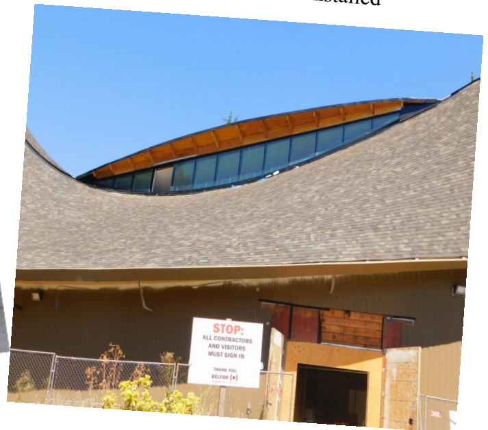
Eyebrow Glass Installed
